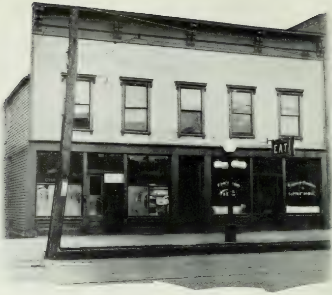
ROOT'S OFFICE AT LYONS Over Restaurant at Right
